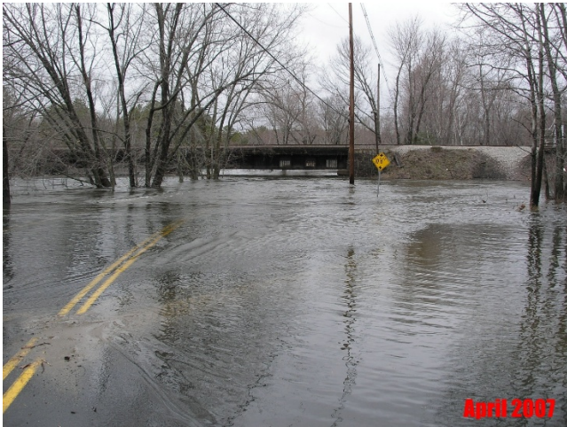
Macpherson Road at Railroad Bridge during flood event
