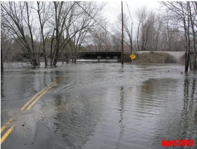
MACPHERSON ROAD AT RAILROAD BRIDGE VIEW NORTH
