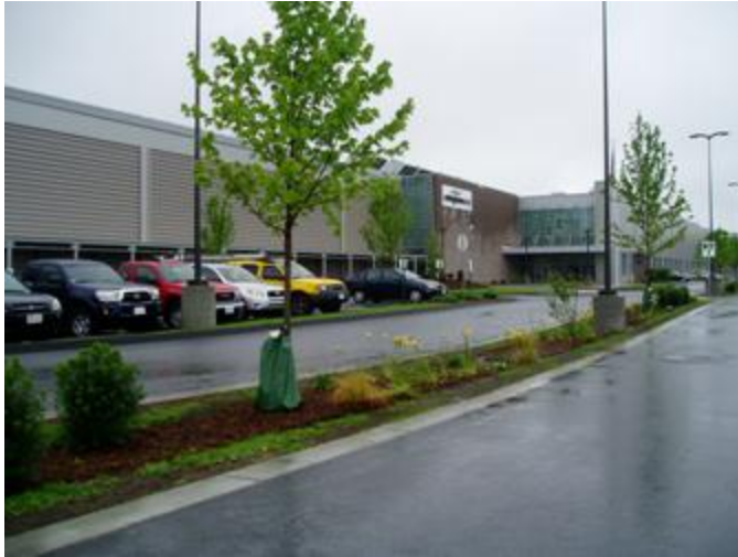
Evergreen Solar bio-filtration landscape islands
