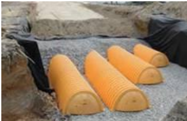
Devens Common underground infiltration systems
