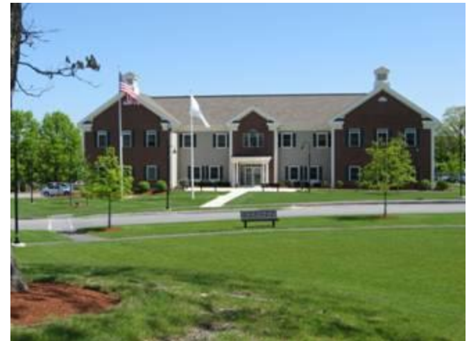
Devens Common cisterns collecting roof runoff
